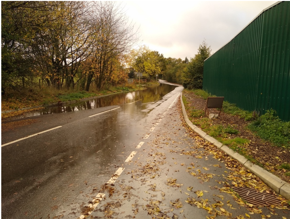
Figure 14.1. Photograph of flooding on Chesham Lane where the west entrance to the site is proposed.
