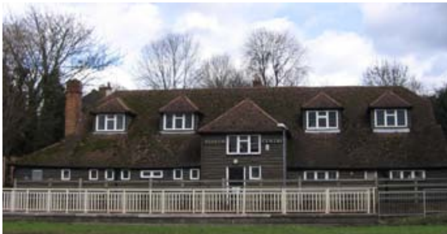
Tithe Barn at the Greyhound roundabout with the entrance to the subway decorated by members of the Youth Club
