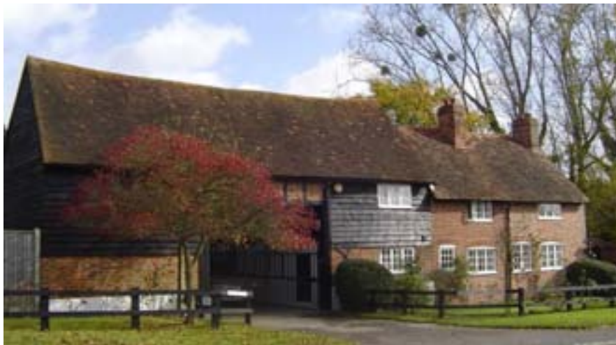
A variety of building styles are featured in this house at Mopes Farm
